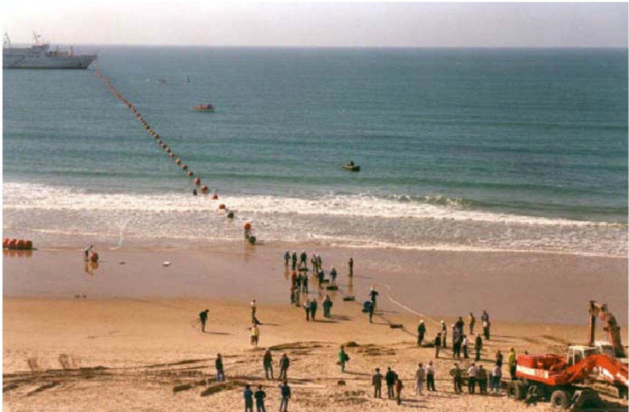
Figure 20: Coastal Landing of Buoyed Cable
